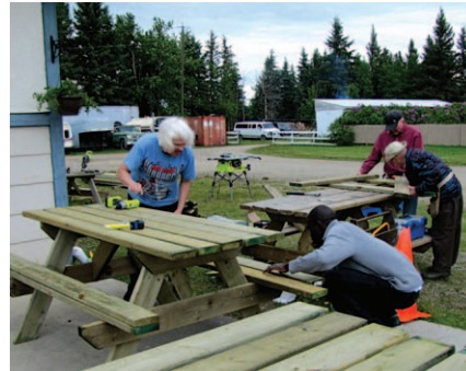
Building picnic tables for Foothills Camp.
