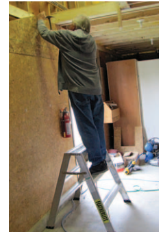
Installing wall board.
