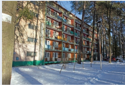
Dilapidated summer resort, home for the family.
