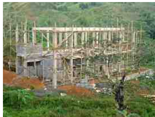
The latest picture we have of the new Dorm/Kitchen building being built at the Philippine Deaf school
